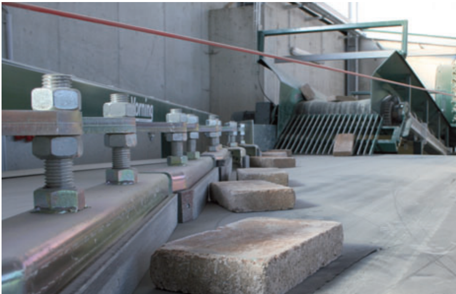
The Organizer arranges the concrete blocks in a longitudinal direction
